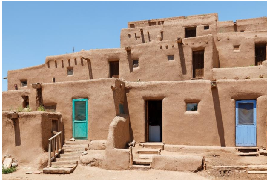
Figure 4.4: An adobe dwelling made from earth bricks and a small amount of wood
