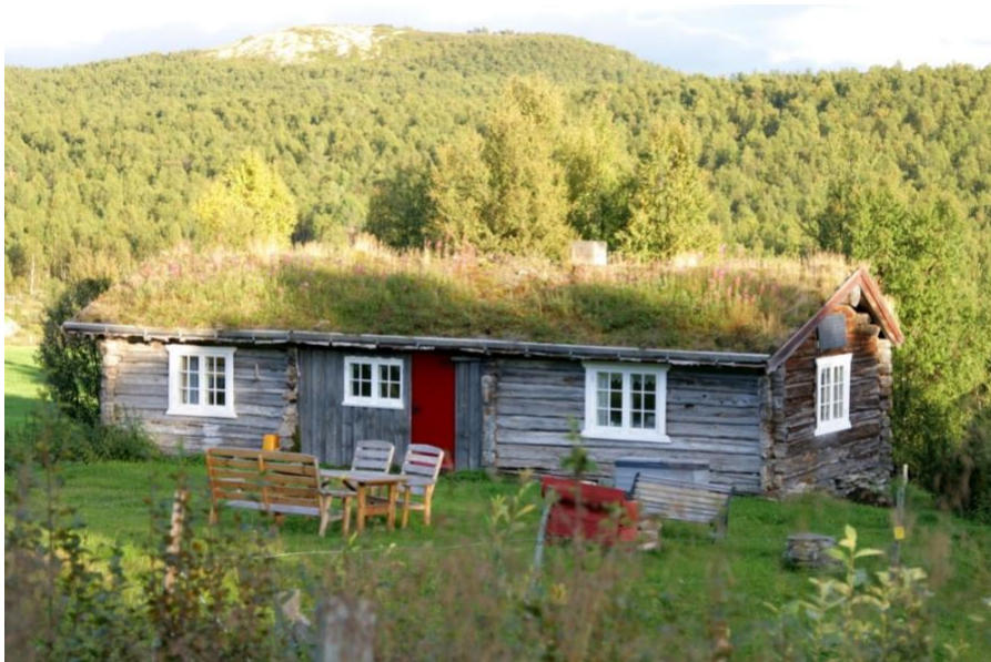
Figure 4.2: A timber house with a sod grass roof
