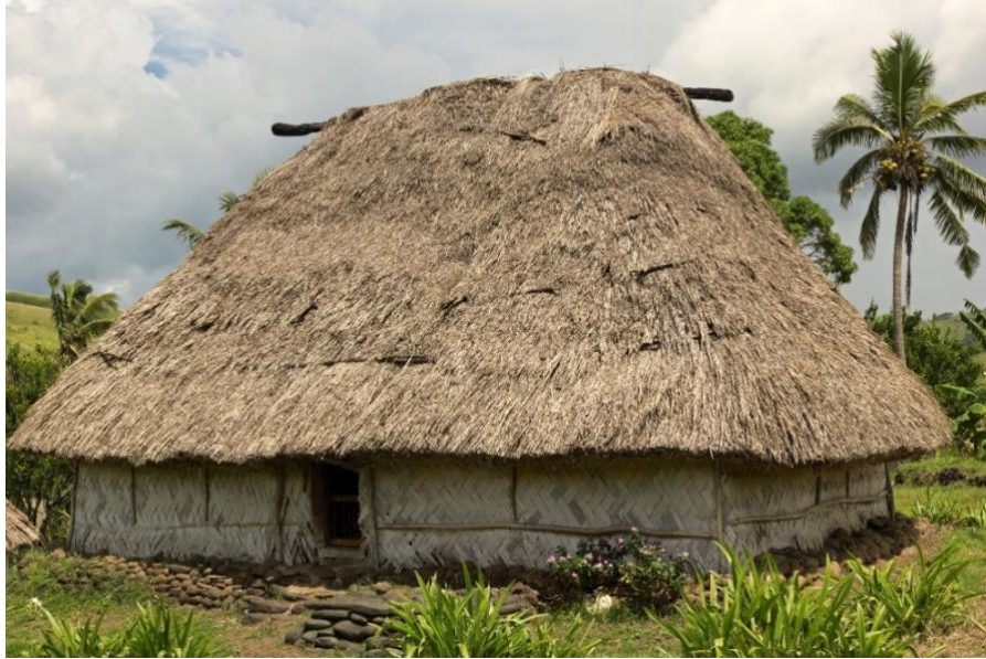
Figure 4.1: A bure with strong wood corner posts, walls of woven mats, and a grass thatch roof
