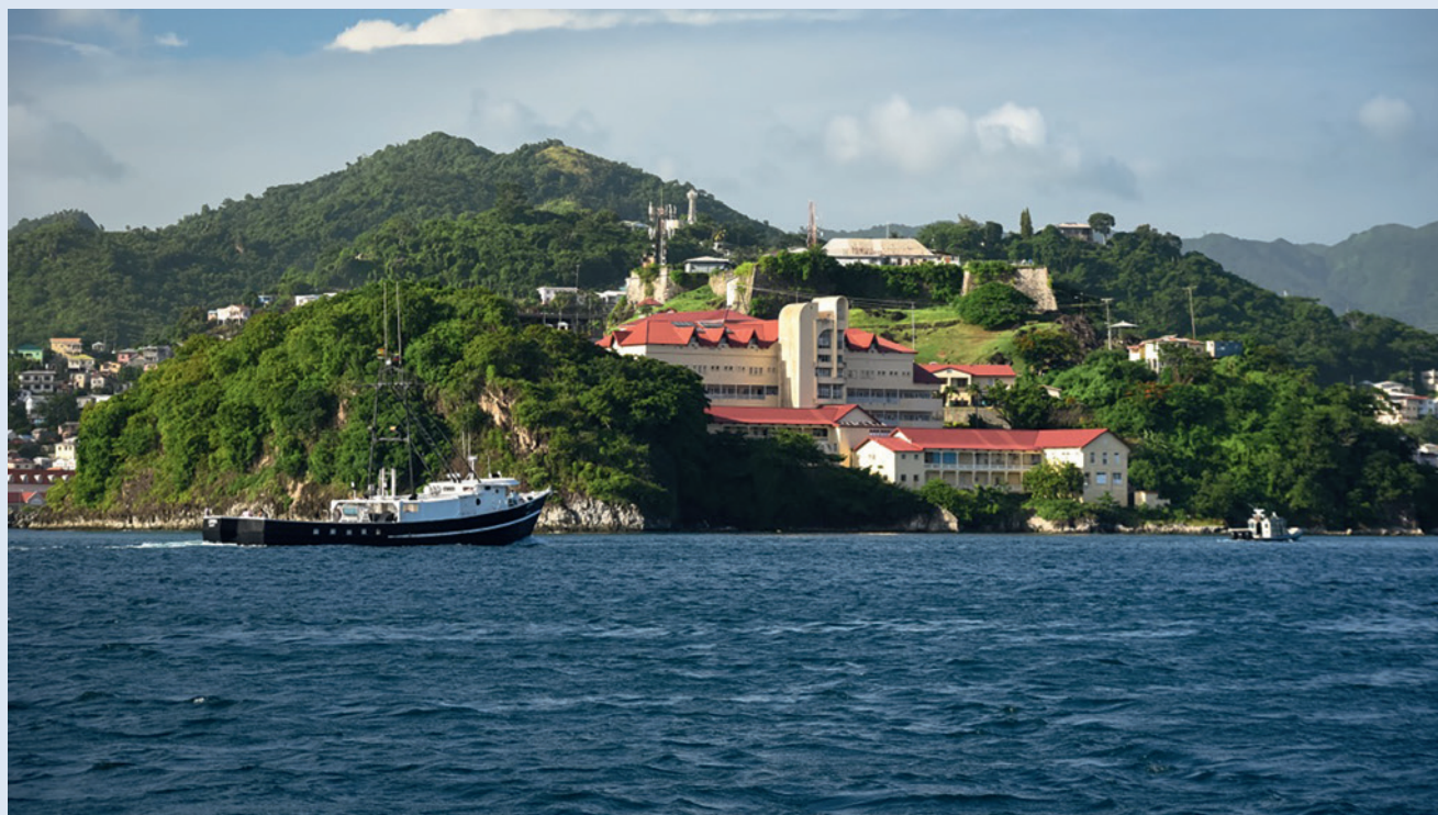
Figure CS 6.2 St. George's General Hospital, Grenada (photograph: Martin Forde).
